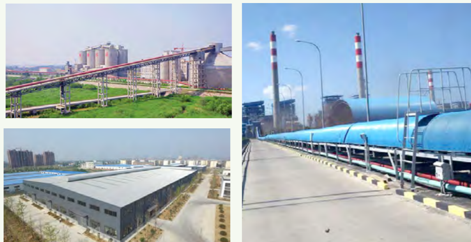
Conveying equipment, steel structure
